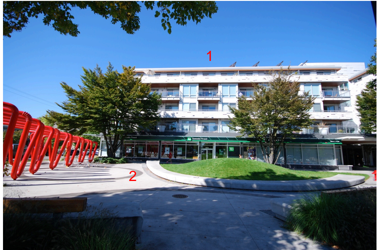
View of the southern end of the development across the pocket park.
