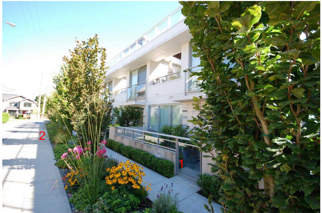
View south showing the townhouses facing the rear lane.
